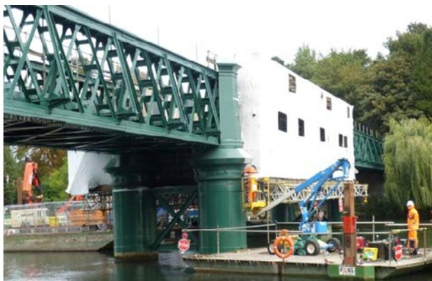
WTN/P/01/07 Encapsulated central span serviced by floating craft
