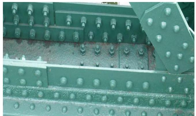
WTN/P/01/09 View of typical rivet replacement by high tensile bolts and like-for-like splice plates to restore an area where there has been a loss of section due to extensive corrosion of the bottom chord of the trusses.
