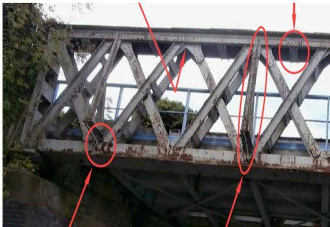
WTN/P/01/04 Bottom chord of trusses were particularly corroded prior to re-painting
