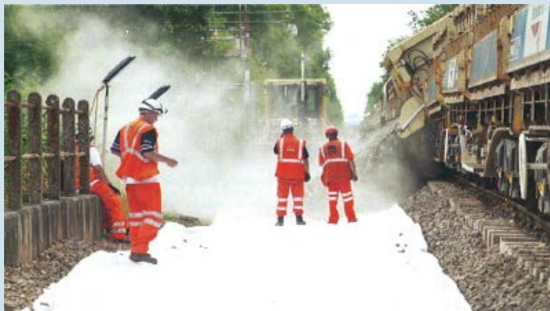
Mind the dust: ballast is dropped at Minety on 20 August 2013. M. John Stretton
