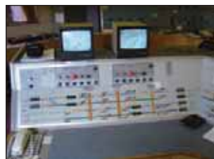
Figure 7 The level crossing control panel mimics the order of the crossings on the rail infrastructure.
