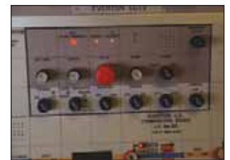
Figure 9 The order of the closing procedure control buttons require the signaller to double check the crossing is clear prior to completing the closing
