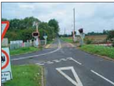
Figure 30 06: two road junctions cross before leading to Bainton Green crossing. The complexity of this junction leads to vehicle drivers having to focus on a variety of different information cues, especially during rush-hours when this is used as a shortcut route.
