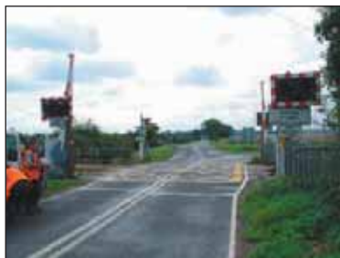
Figure 31 24: Bainton Green is a half barrier crossing. Zig-zagging has been observed by locals.
