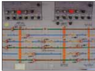
Figure 11 The level crossing control panel mimics the order of the crossings on the rail infrastructure.
