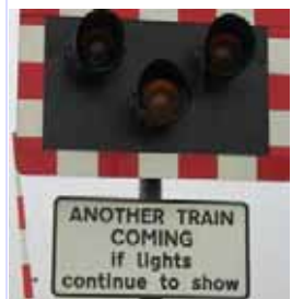
The sign 'ANOTHER TRAIN COMING if lights continue to show' is positioned underneath the wigwag lights.
