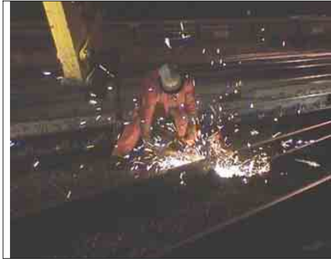
Figure 37. A rail disc cutter in use.
