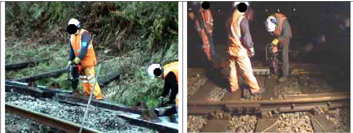
Figure 34. Working postures during use of the same model of nut-runner.
