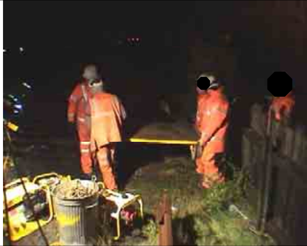
(a) Four person carry of a large rail trolley (124kg)
