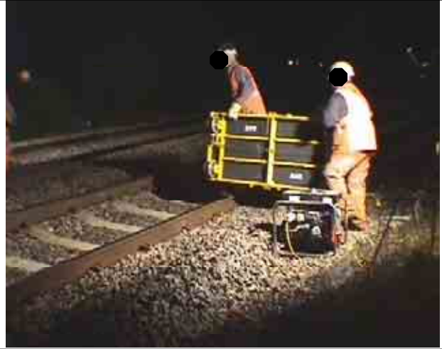
(b) Two person carry of a small rail trolley (54kg)
