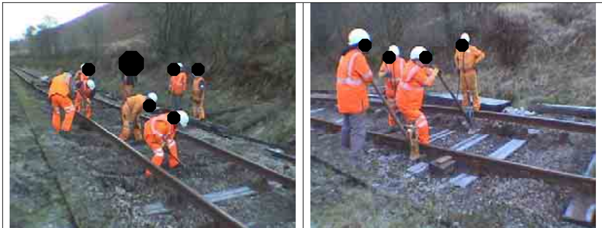
Figure 18(a) Preparatory digging .
