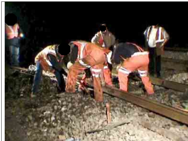
Figure 24. Four workers dragging sleeper out from under rails.
