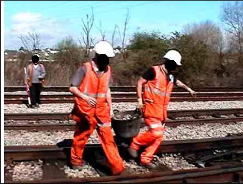
Figure 46. A typical carrying operation when moving ballast (with 50kg bucket load)
