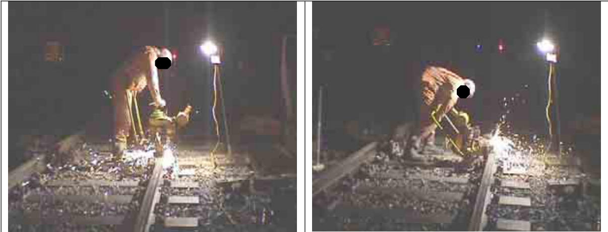
Figure 31. Two typical postures illustrating the range of trunk flexion involved in the grinding operation.
