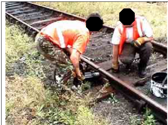
Figure 35. Nut runner used to fasten Fishplate bolts.
