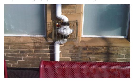
In June 2011 the results of monitoring the effectiveness of the radon pumps at Shipley showed a level of 110 Bq/m<sup>3</sup>, 290 Bq/m<sup>3</sup> below the actionable limit.
