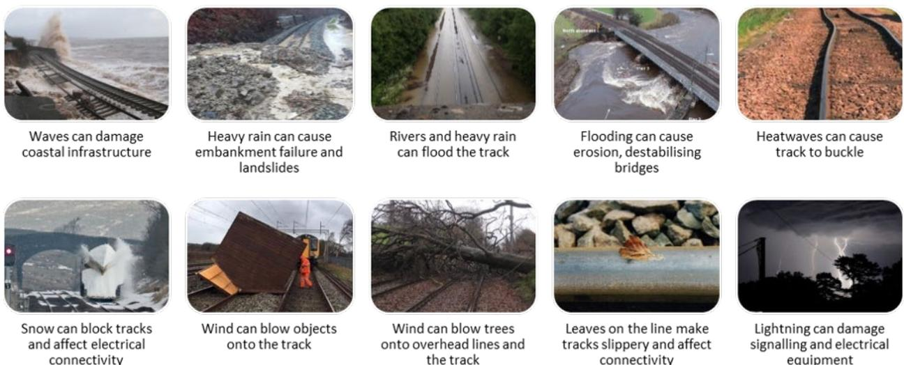
**Figure 1:** Impact of weather on Network Rail Assets (source: [Network Rail](#)).
