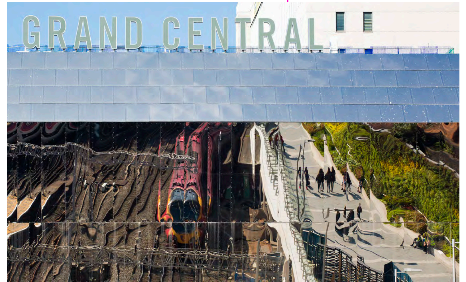
Green wall reflected in cladding at Birmingham New Street Station. Image ©2022 Network Rail.
