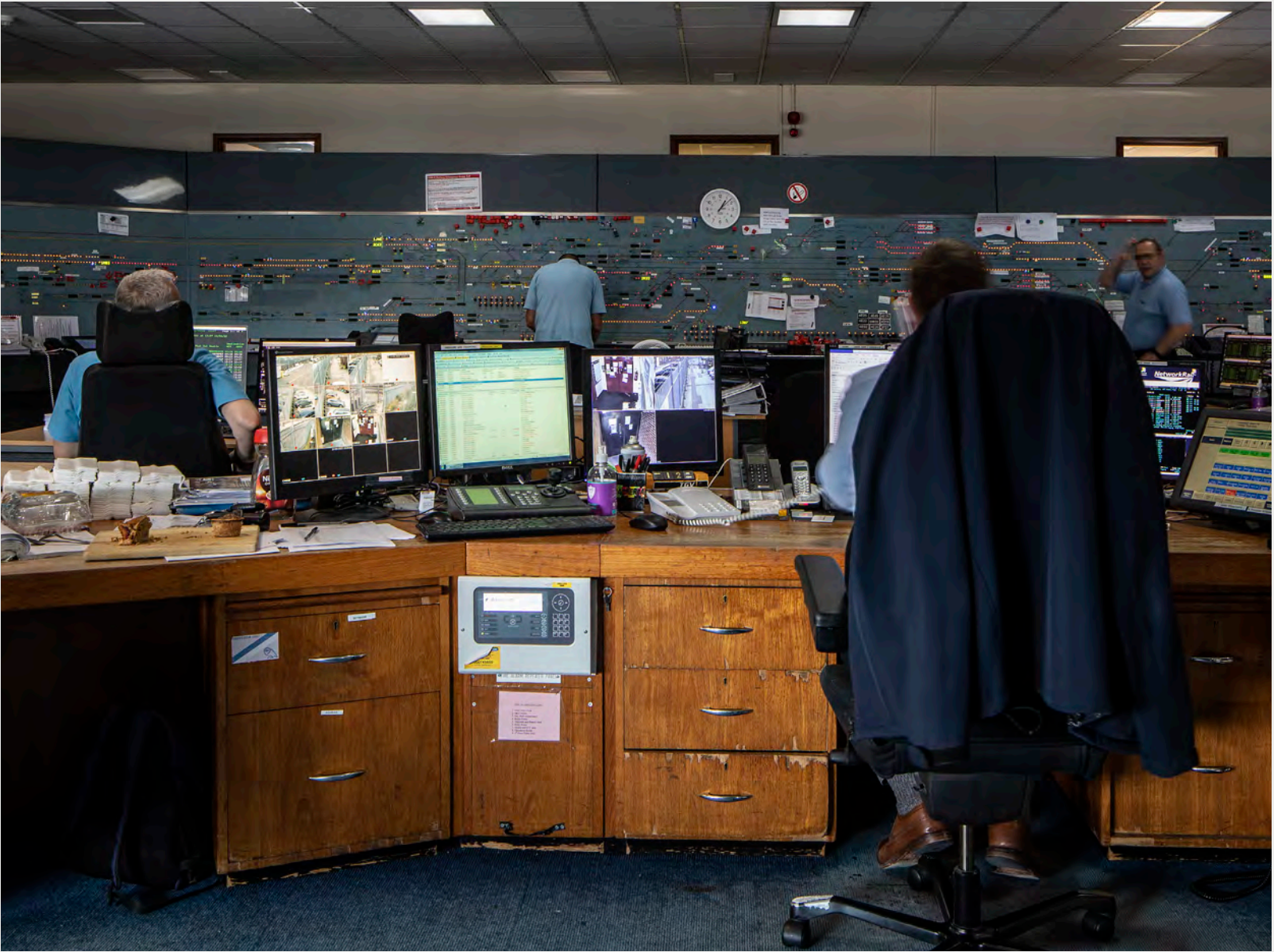
Doncaster control room. Image © Adelina Iliev.
