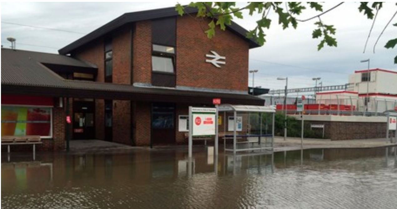
Figure 2: Network Rail asset in flooded area
