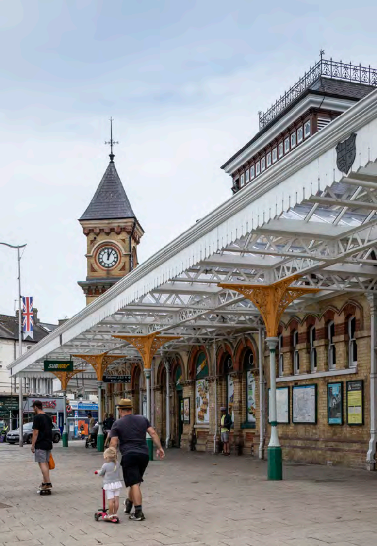
Renovation and upgrading of Eastbourne Station. Image (left) © Adelina Iliev. Image (above) ©Adelina Iliev.
