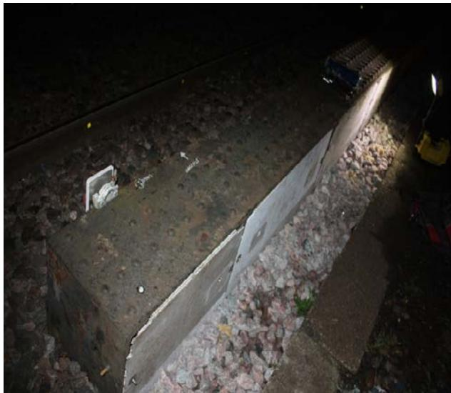
WEX/HCE/02/03 – centre main girder with inspection hatches at either side of the GRP ballast plate
