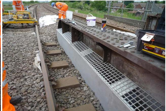
LNE/HCE/01/05 – typical GRP ballast board retaining proposed for site (installed around web stiffeners)
