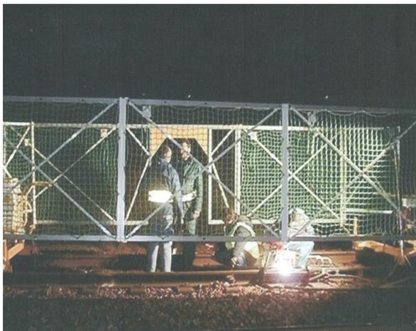
**Weld repairing inside a Geismar barrier system**
